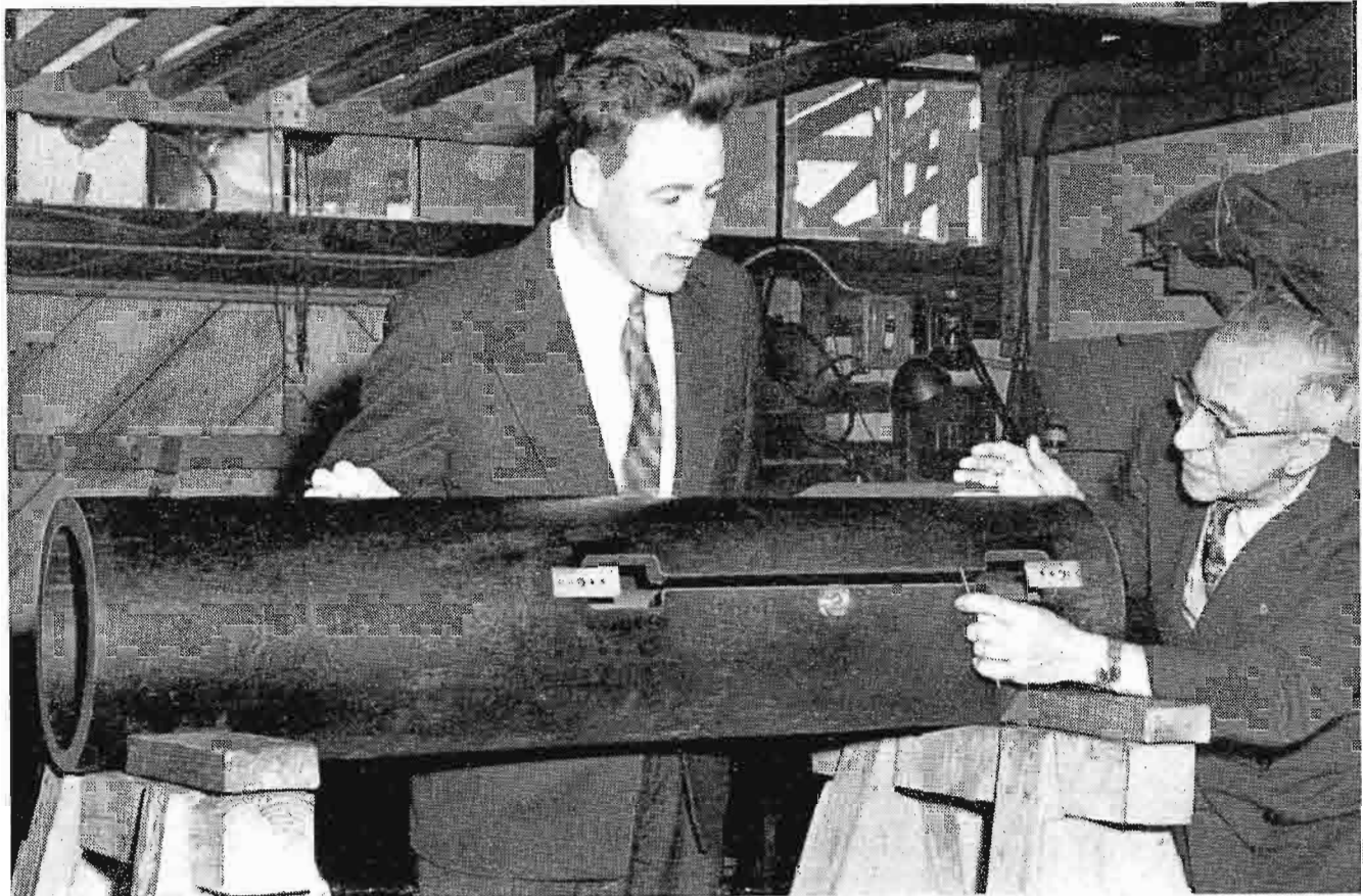
FIG. 7. Final inductively tuned slots for a gain of 9 antenna on 10 \frac{3}{4} inch diameter pole section being inspected by the authors, Matti S. Siukola (left) and George A. Kumpf.
