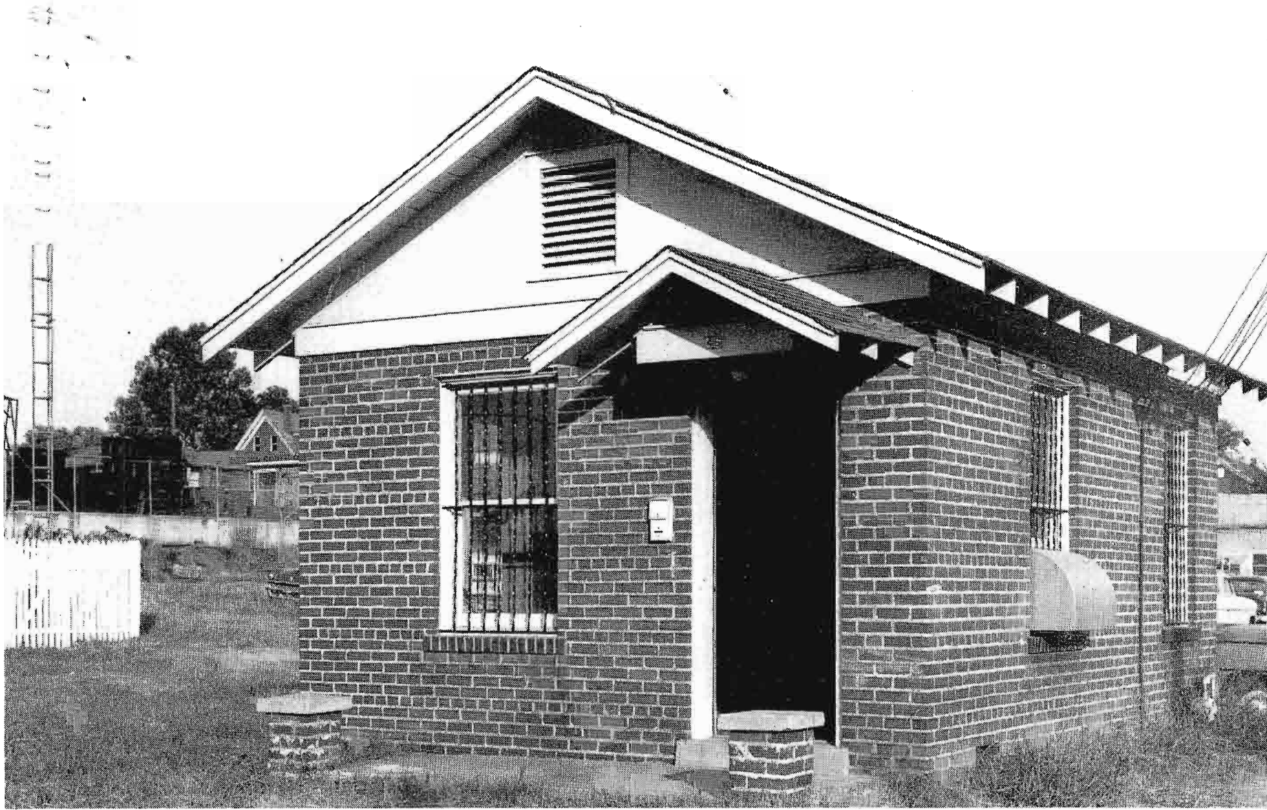
FIG. 8. Transmitter building contains a remotely controlled RCA B1A-1M AM Transmitter.
